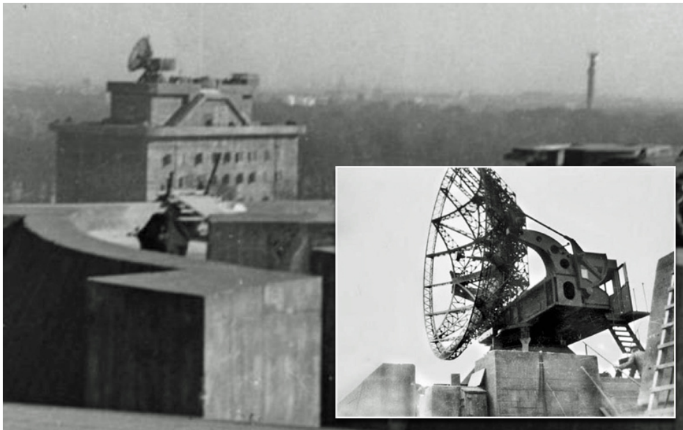
Photo 09: The Zoo control tower in the background, seen from the G-tower. Inserted the Giant Würzburg radar that could be lowered into a 12 meter deep internal shaft as enemy planes approached.
