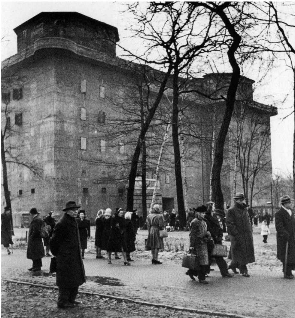
Photo 12: Civilians flocking outside the shelter, apparently after the all-clear has been sounded. Date unknown, but must be while conditions were still tolerable. 27 mm and 20 mm guns are not immediately visible which could indicate a postwar photo, but why then would so many be congregating there?
