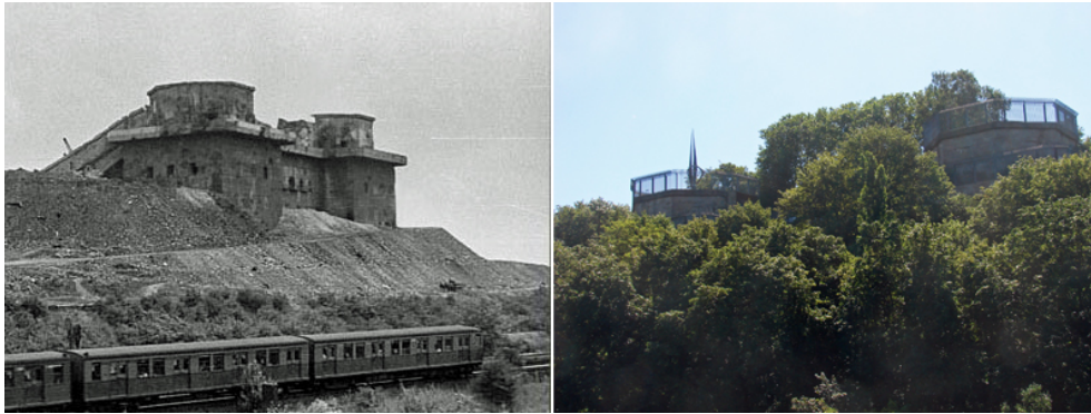
Photo 22: Humboldthain towers were only partly demolished and the G-tower is accessible today during organized tours.
