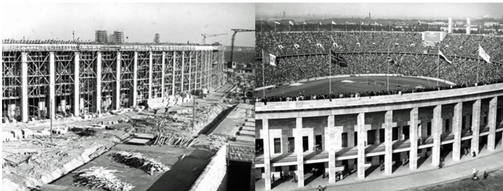
Photo: Olympic Stadium during construction and in 1936. All in all it looks pretty much the same today.
