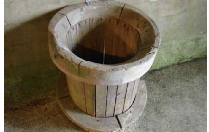
Original wooden chute for spent shells leading to a basement chamber
