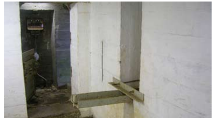
Chute from ammo storage room to gun.
